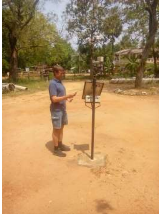
Figure 11: Pole structure leaning to the right in UO_ATHURUWELA
