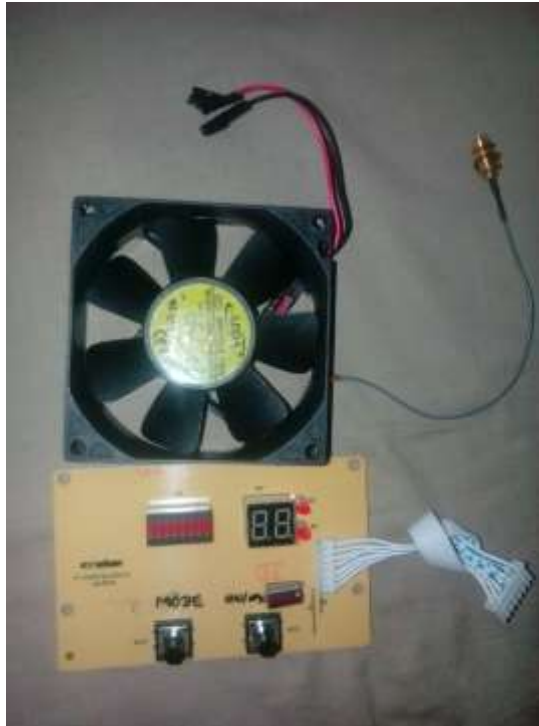
Figure 13: broken fan, rusted aerial cable and misbehaving solar controller interface
