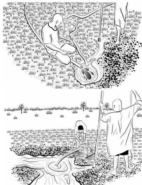
Connect pump for jetting with drilling pipe, lift water into the mud pit and ensure tight connections
