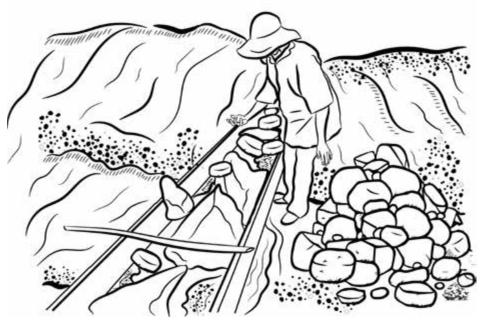
Construction of stone boulder embankment dam across a stream
