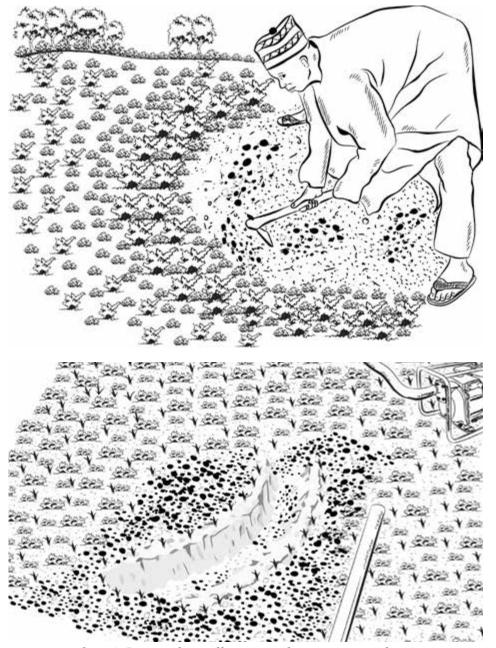
Step 2: Locate the well point and construct mud pit
