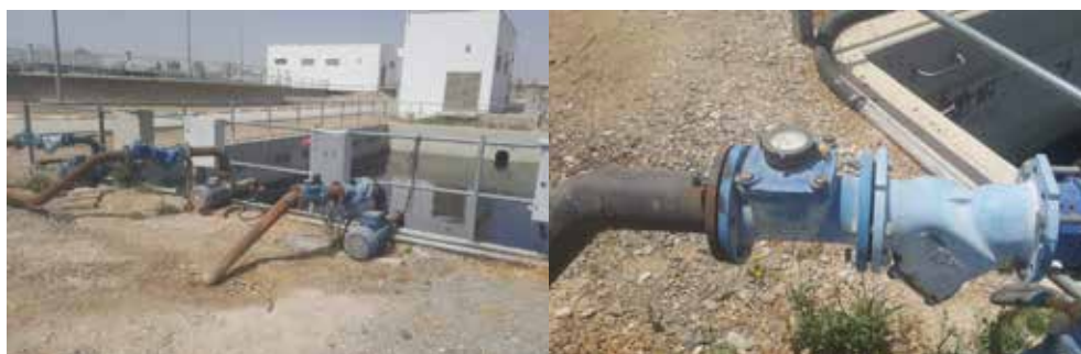
IMAGE 5.3 Effluent storage and irrigation tank and the effluent pumps and the flow meters at Jericho WWTP. Photos: I Abu Seiba.
