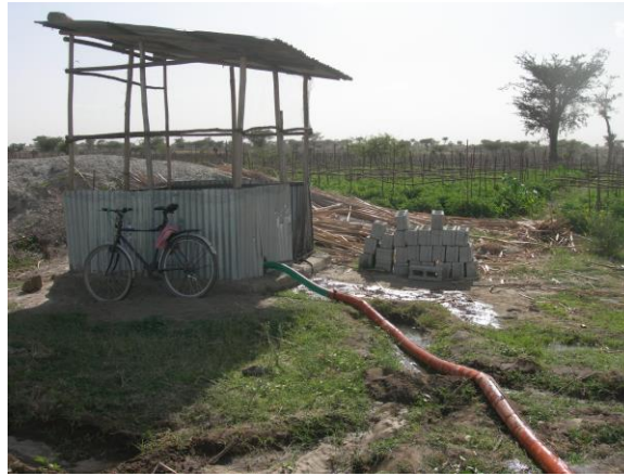
An irrigation pump house constructed for a 12-member WUA, near the town of Meki, Ethiopia
