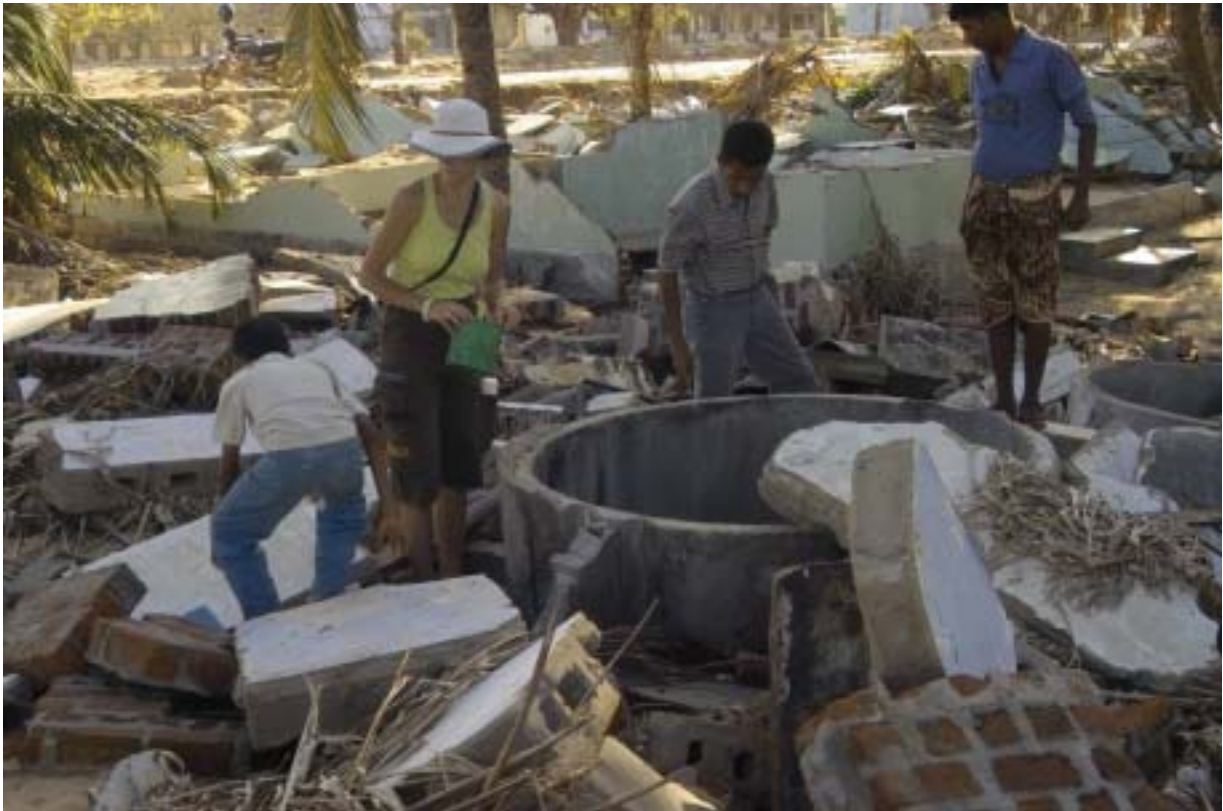
Figure 15. Initial well salinity monitoring in Maruthumunai, end of January, 2005
