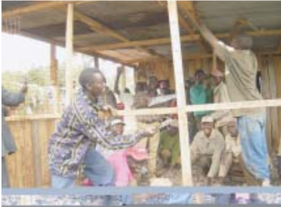
Members of the Tri-Hills SHG build their shed
