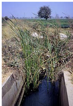
Fred Pearce Canals carrying water from the Kano Irrigation Project in Nigeria are clogged with weeds.
