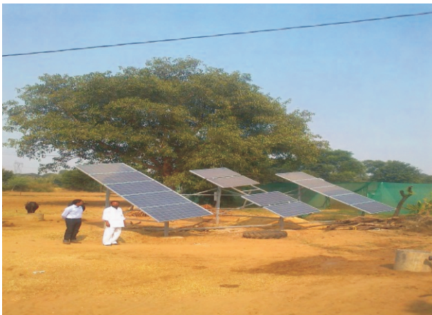
Picture 2- A 2200 wp Solar Pump Array
