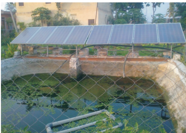
Picture 2- A 2200 wp Solar Pump Array
