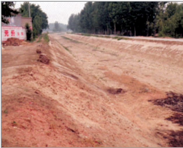
Figure 2 A CC lined branch canal
