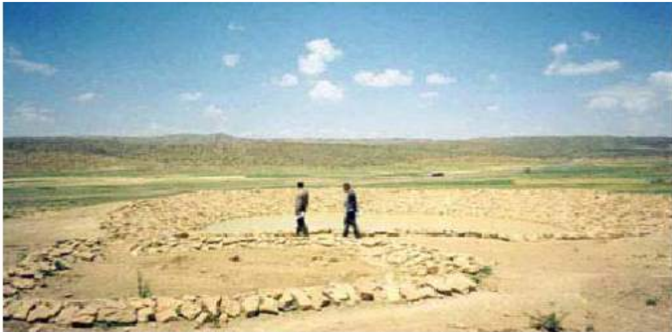
Rapid siltation: Full silt trap due to lack of watershed treatment, Geteb Dawru watershed (photo H.Rämi, UN-OCHA, Oct 03)
