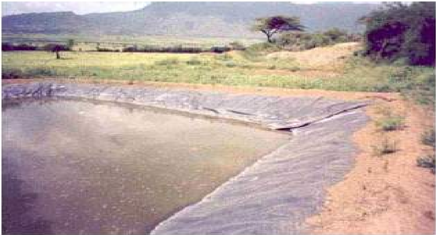
Cheaper than concrete: Plastic lined pond Alamata
