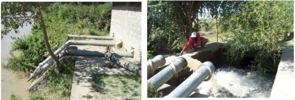
Fig 3.1 Irrigation water abstraction at Batu Degaga
