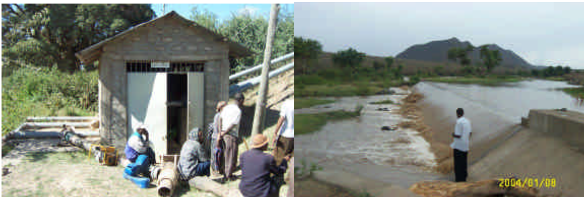
Fig H-7. Pump house at Batu Degaga and excess water diverted flows back to the Awash River over the diversion weir
