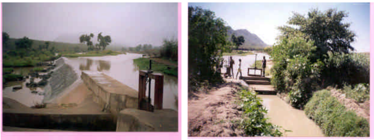
Fig 3.2 Diversion weir and the main canal at Doni irrigation project
