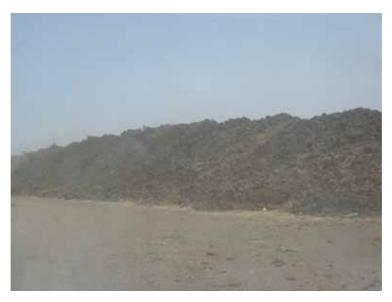
FIGURE 29. Sedimentation challenges in canals of 80 km Meana to Rahad conveyance. Note the canal is behind the pile of dredged sediment (photo credit: Seleshi B. Awulachew).
