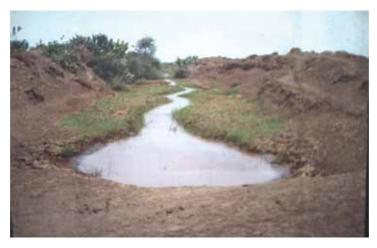
FIGURE 28. Sedimentation problem in the Gezira scheme canalization system (photo credit: Abdella A. Ahmed).
