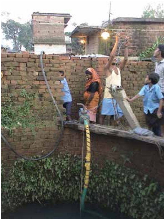
Farmers in Jharkhand State, India tap into local electricity lines to power their pumps.
