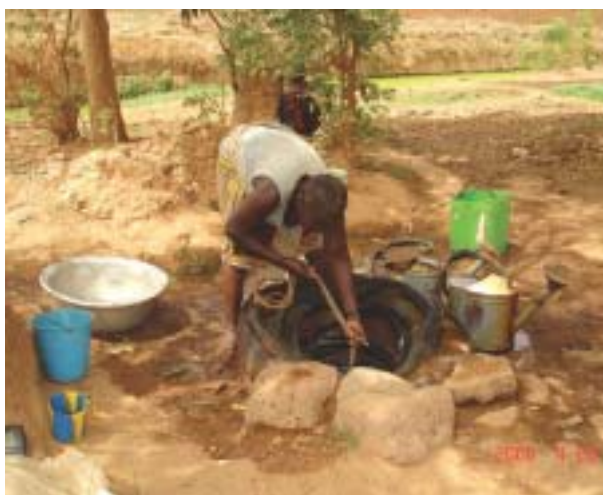
Vegetable farmer lifting water from a well stabilized with car tyres
