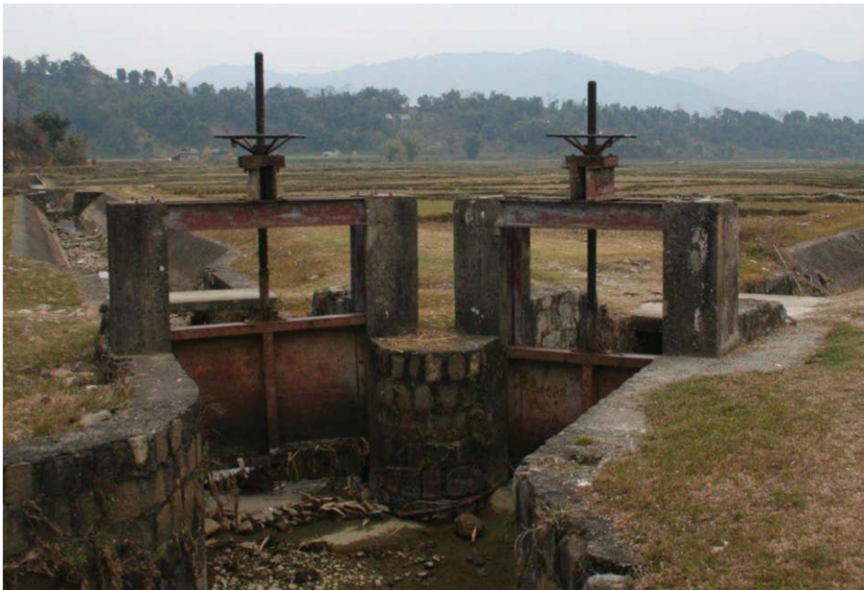
Control gates divert water to two different water user groups when they are planting (Photo credit: Karen Conniff, IWMI).
