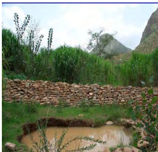
Figure 6. Biophysical gully treatment
