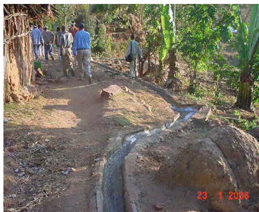
Figure 3. Canal reinforced by cemented wall to reduce water loss, at Metta woreda, East Haraghe Zone
