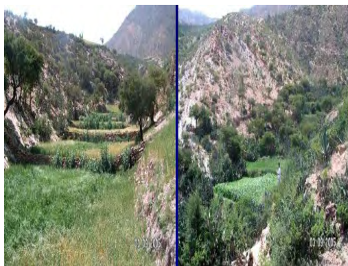
Figure 3. Traditional sediment storage dams
