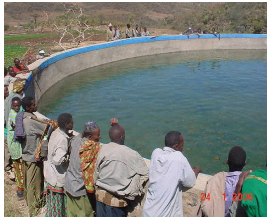
Figure 1. Water storage constructed at high elevation at Goro Gutu woreda, East Haraghe Zone
