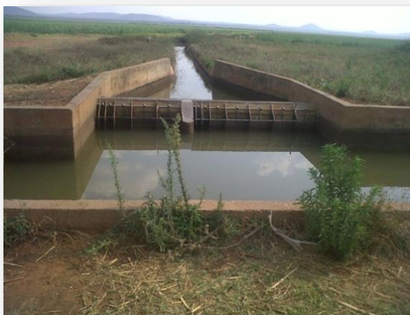
Left: Water intake structure
