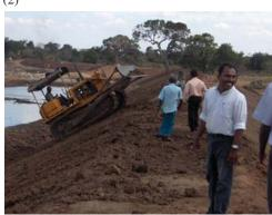
Figure 3. Contour lining for soil water conservation bunds.
