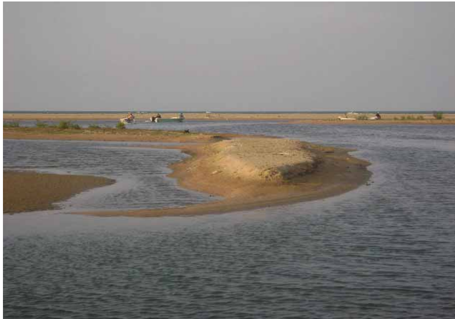
Figure 42. Artificial opening of the lagoon to allow for movement of marine fishing crafts - Kappaladi Lagoon, Chilaw.
