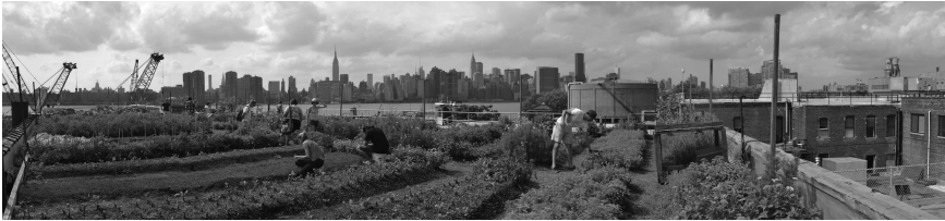
FIGURE 4.9 Eagle Street Rooftop Farm, Queens, New York (USA): one of several rooftop farming initiatives in North America
