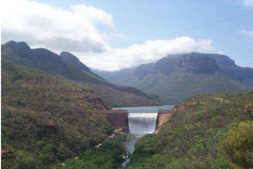
Blyde river dam in January (credit photo IWMI-SA)
