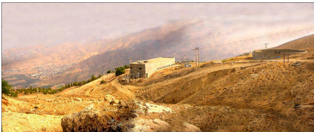
Figure 5-39. The pumping station and a basin of the Zai-Dabouq conveyor pumping water from the Jordan Valley to Amman (Papin, 2007)
