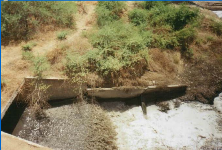
Treated sewage from Vasna STP meets Sabarmati near Gyaspur
