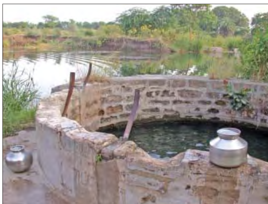
Figure 10. Open well water level is up to the ground level recharged by water harvesting structure (WHS).
