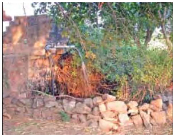
Figure. 21. Bore water is pumped into open well and used for irrigation.
