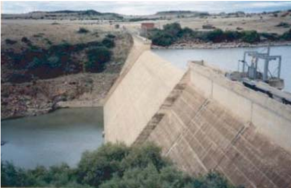
FIGURE 12. Partial view of the downstream side of Rustfontein Dam.
