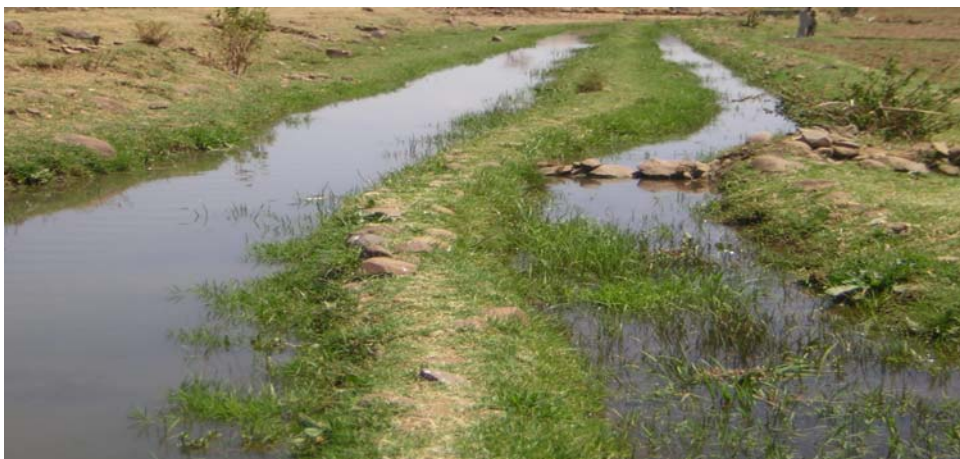
Fig.3.10 Ponding water with very small speed in secondary canal, Haiba
