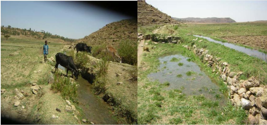
Fig.3.8 Livestock interference and overfilling of canals result in wastage of water and water logging
