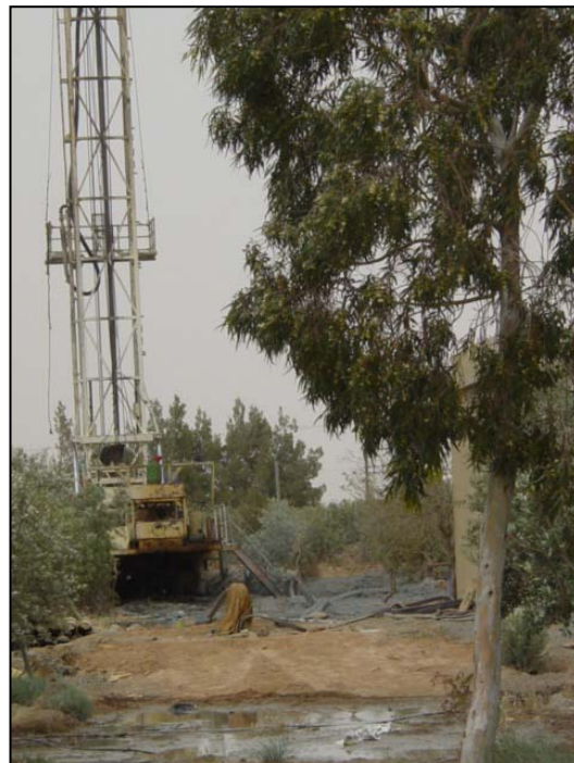
Picture 3 & 4: Drilling well
